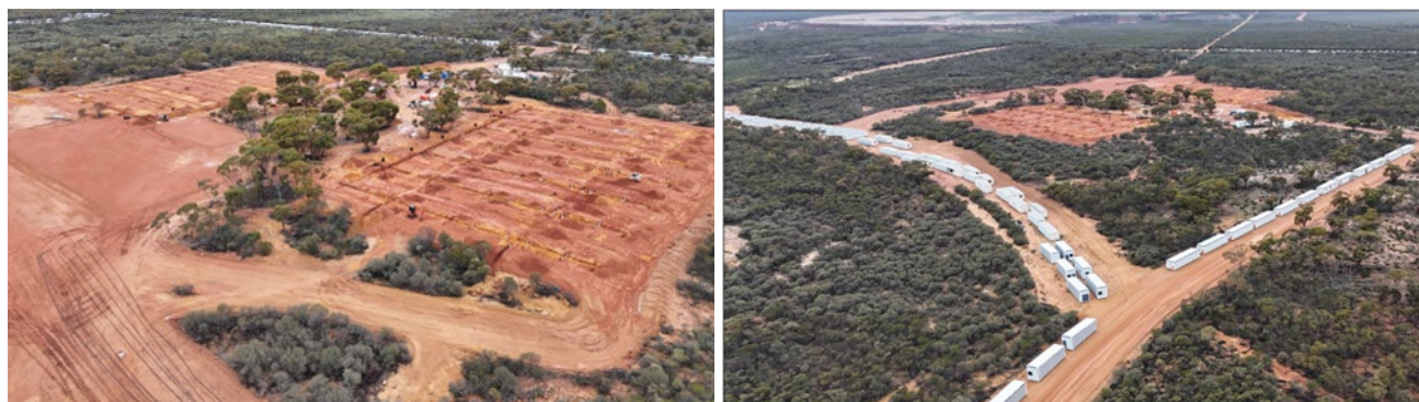
Mt Gibson Gold Project – accommodation village installation
